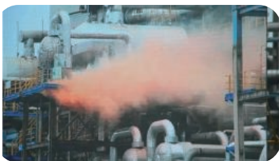
Onsite Emergency Detection
