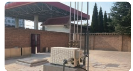
Oil and Gas Recycle Site Inspection
